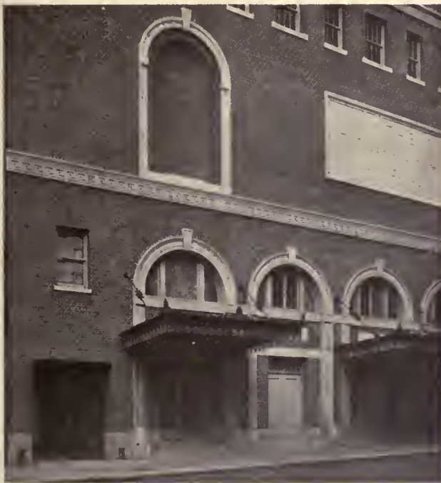
ENTRANCE DETAIL THE TOWN HALL, NEW YORK CITY McKIM, MEAD & WHITE, ARCHITECTS
